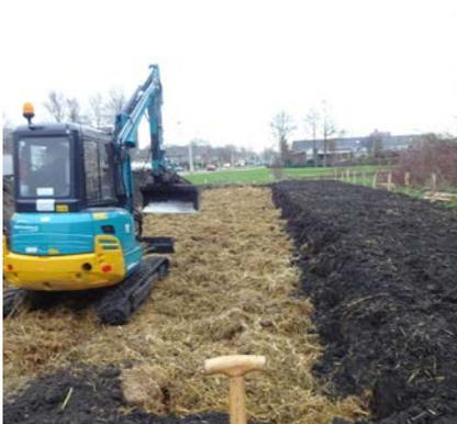
**5.** Mix the soil supplements through the dirt using the excavator.
