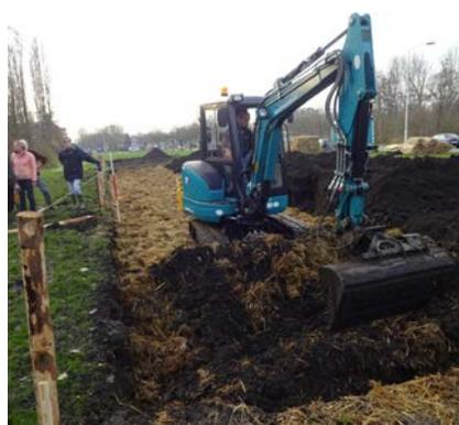
**6.** Now pour the rest of the excavated dirt back into the trench, and mix in the other half of the soil supplements.
