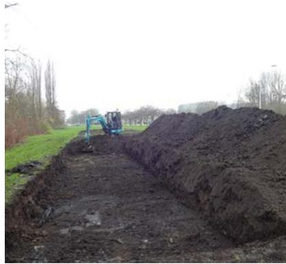
**2.** Excavate the length and width of the Tiny Forest down to 1 meter deep, and place the excavated dirt next to the trench.
